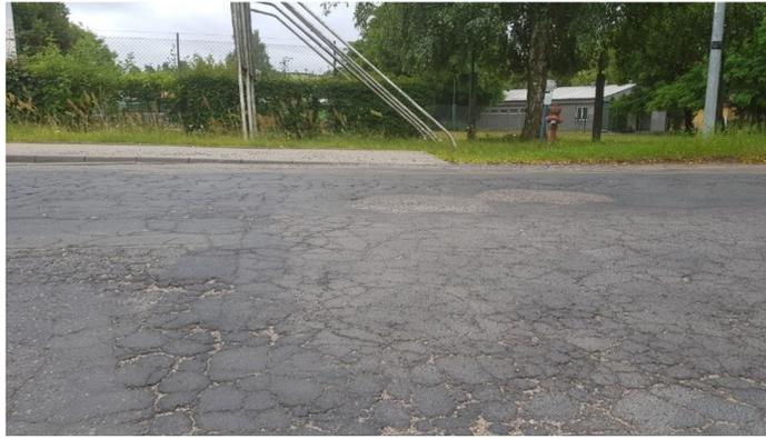
**Figure 9.** Worn road surface (WRS) used in research, photographed from the point of view of a parked car.
