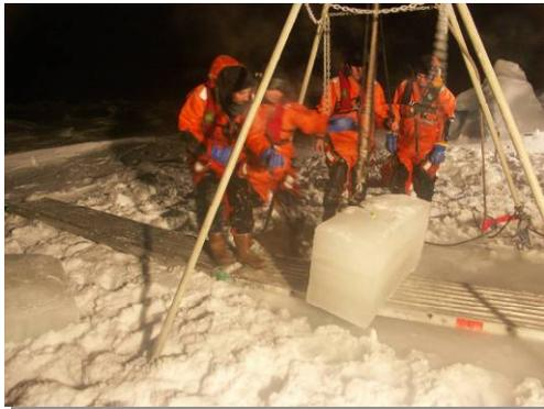
Fig. 17.3: Tripod-pulley-anchor system with aluminium planks to remove the ice blocks from the hole
